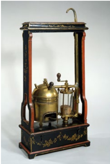
Fire pump MHS 77 Wood, copper, brass, glass, Nollet (?), Paris, 18th century
